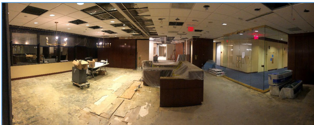
Renovation to the Firm's Fairfax office space in 2021-22
